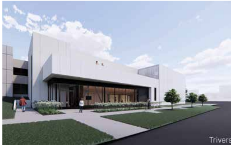
▲ An overall view of the exterior addition at the northwest corner of Kemper Hall. The exterior facade includes several materials including a translucent wall system which will allow natural light into the high-bay training space.
